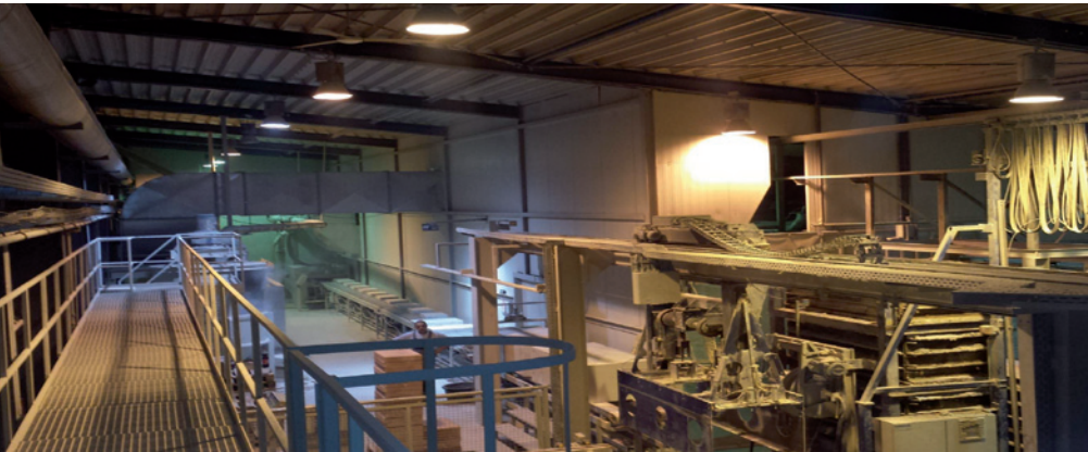
Old Lighting System
