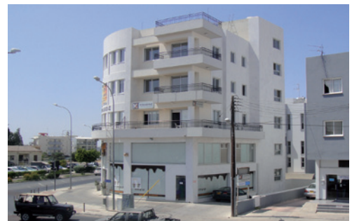
Halloumas House Construction
