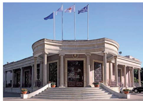
Nicosia Municipality Town Hall Building
